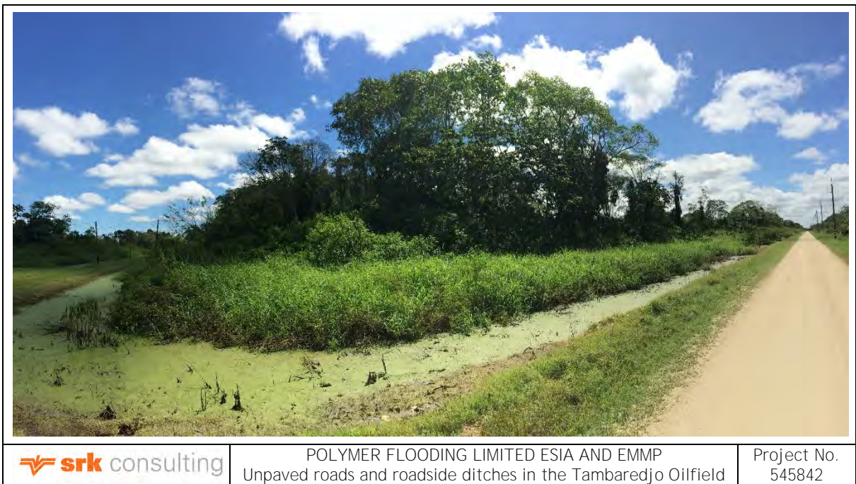
Figure 3-2: Unpaved roads and roadside ditches in the Tambaredjo Oilfield
