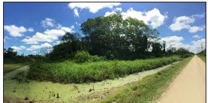
Figure 4: Unpaved road and roadside ditches in the Tambaredjo Oilfield
