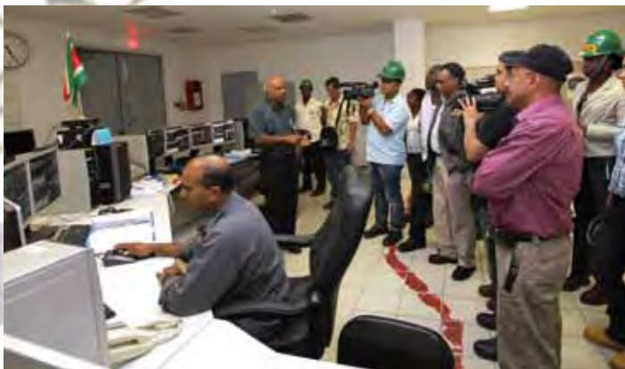
In de controlekamer van de raffinaderij. The control room of the Refinery.
