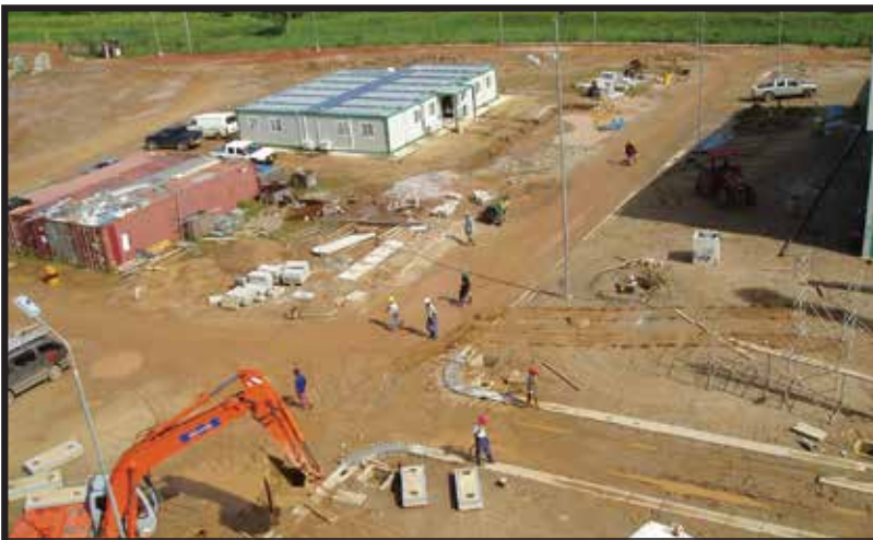
2006 Start bouw SPCS-powerplant. Start construction SPCS powerplant.
