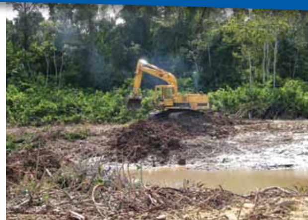
De Gangaram Pandayweg is aan de rivierzijde verhoogd met klei. The river side of the Gangaram Pandayweg has been raised with a clay dam.
