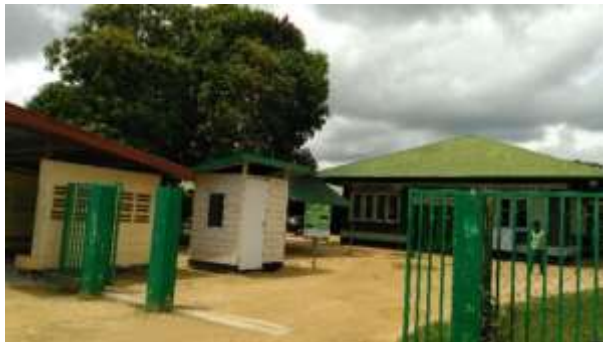
Photo 18: RGD clinic in Totness (km 141)
