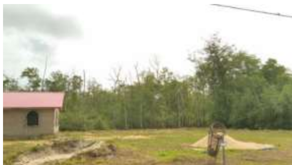
Photo 11: House under construction approx. 120 m south of proposed well location CEP02
