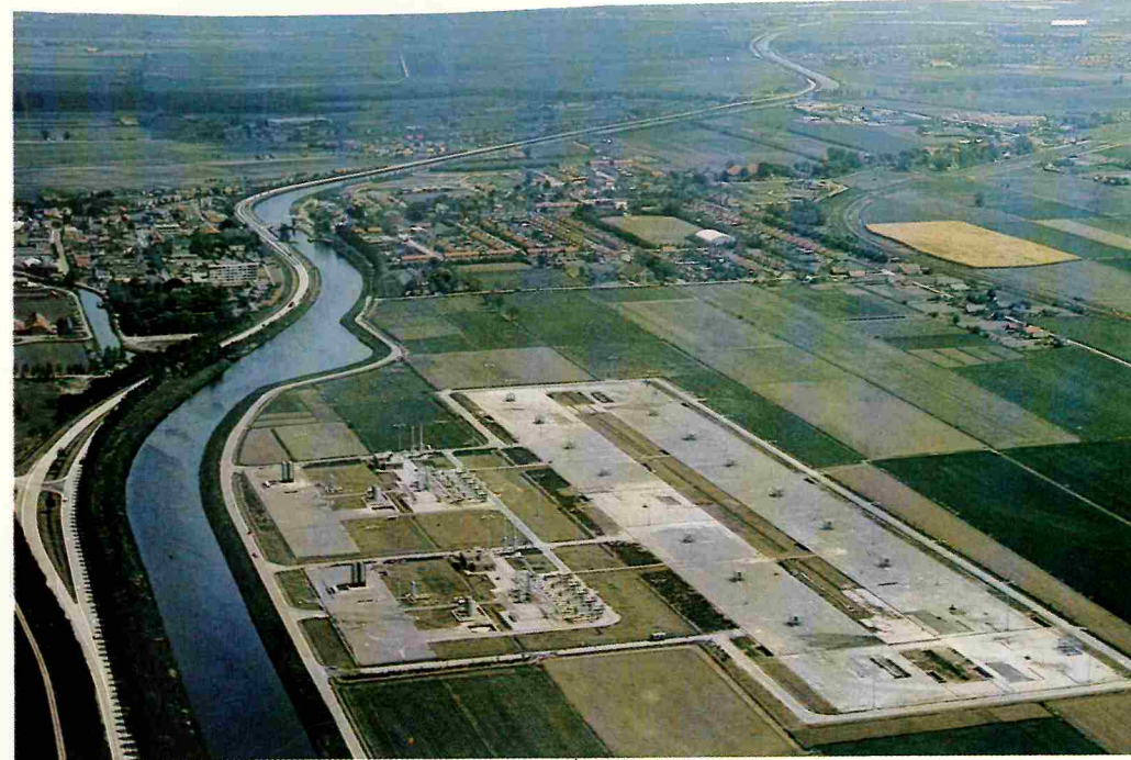
Well cluster "De Eeker" in the Groningen gasfield. The village of Scheemda is in the background.
