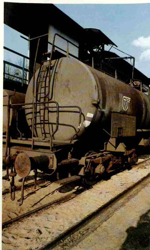
The crude oil shipment station at Schoonebeek.
