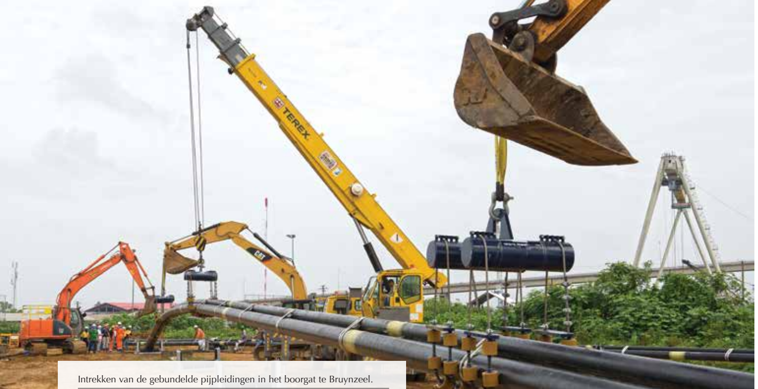
Hauling the bundled pipes in the drill hole at Bruynzeel.
