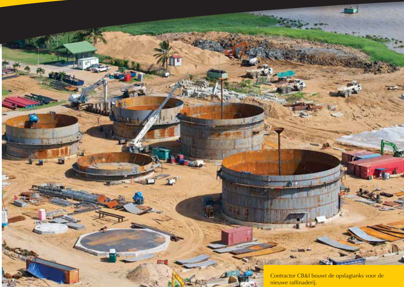
Contractor CB&I constructs the storage tanks for the new refinery.
