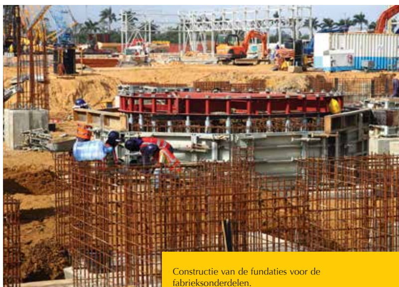
Construction of the fundaments for the factory modules.
