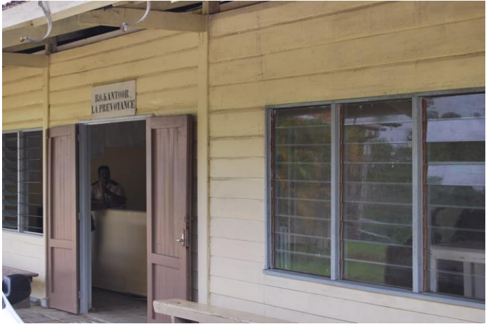
Figure 6. BO Office at La Prevoyance
