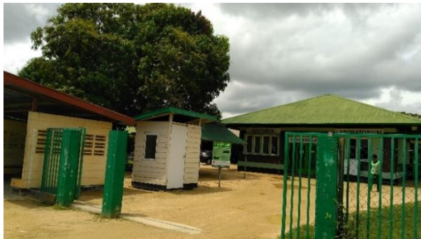
Photo 18: RGD clinic in Totness (km 141)
