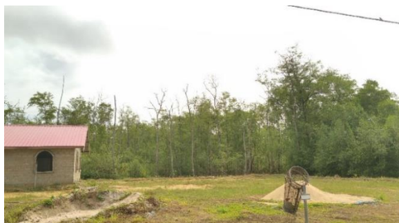
Photo 11: House under construction approx. 120 m south of proposed well location CEP02
