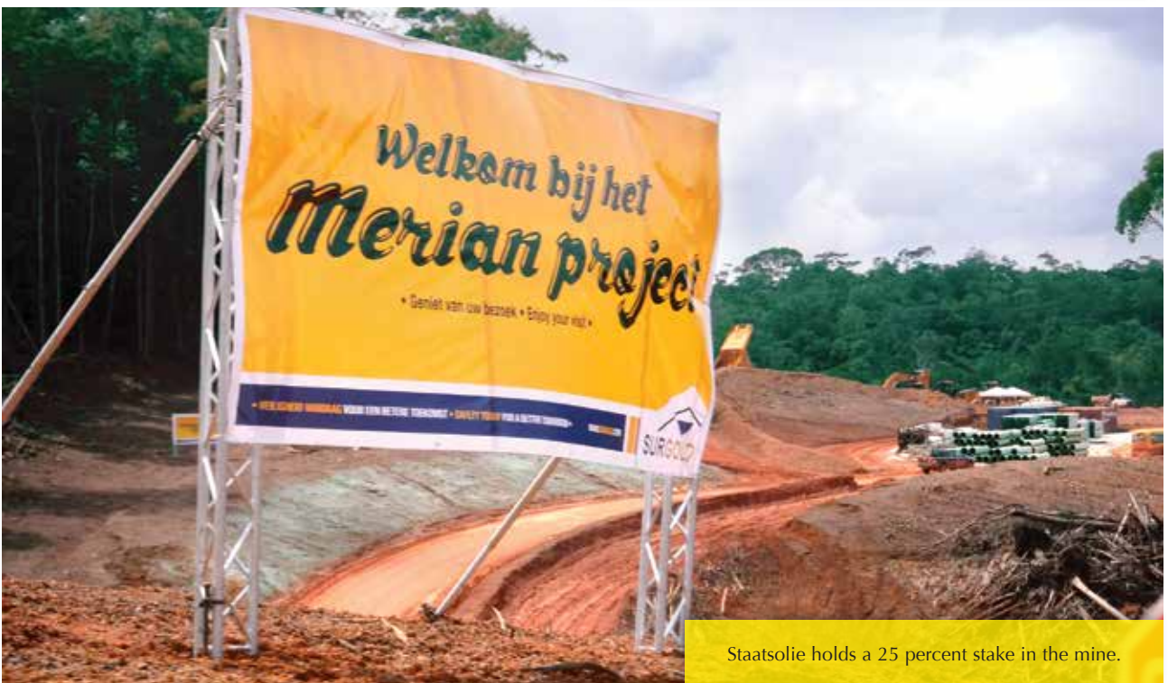
Construction activities at the Merian goldmine in Nassau.
