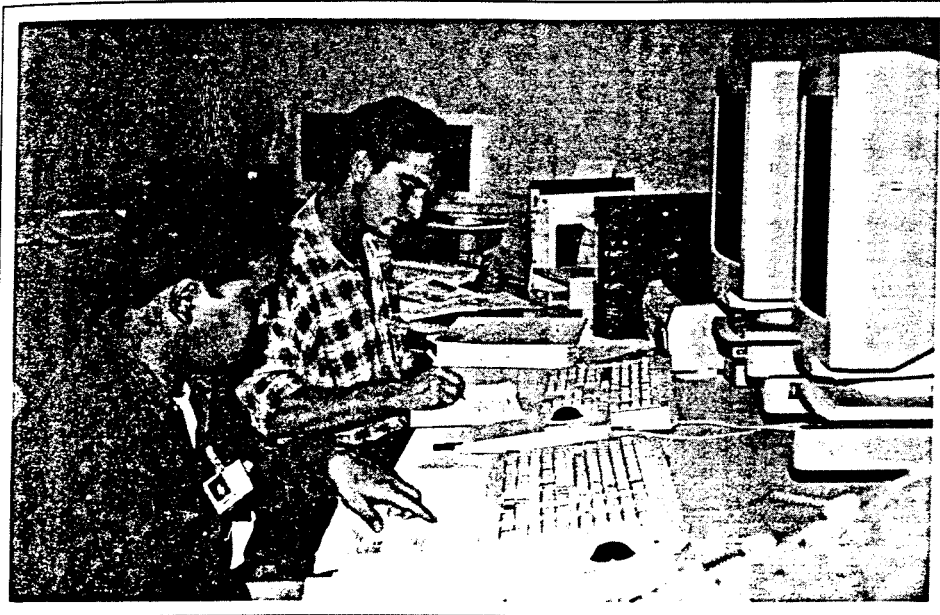
Operator stations in de controlekamer
