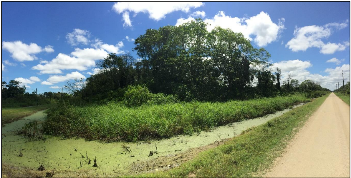
Figure 3-1: Unpaved roads and roadside ditches in the Tambaredjo Oilfield
