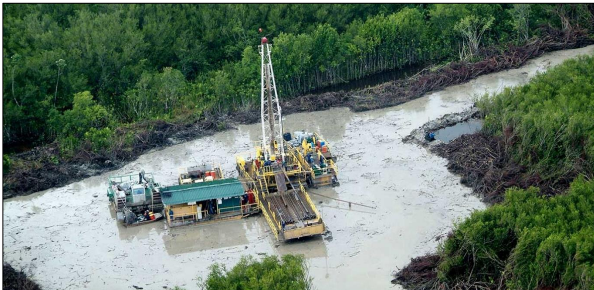
Figure 3-6: Well installation in the Calcutta Oilfield
